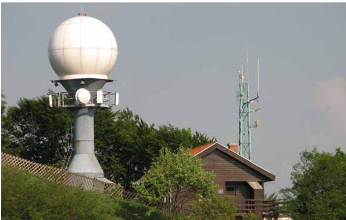
Meteorološki radar na Lisici Meteorological radar station at Lisca
