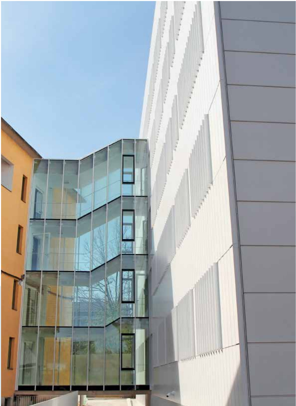
Laboratorijski prizidek Agencije RS za okolje Extension to the laboratory of the Slovenian Environment Agency
